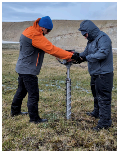
Figure 9. Left photo: Eric and Logan drill into the active layer to install the groundwater well. Right photo: Installing the groundwater well. (CC BY-NC-SA 4.0: W. Ray)
